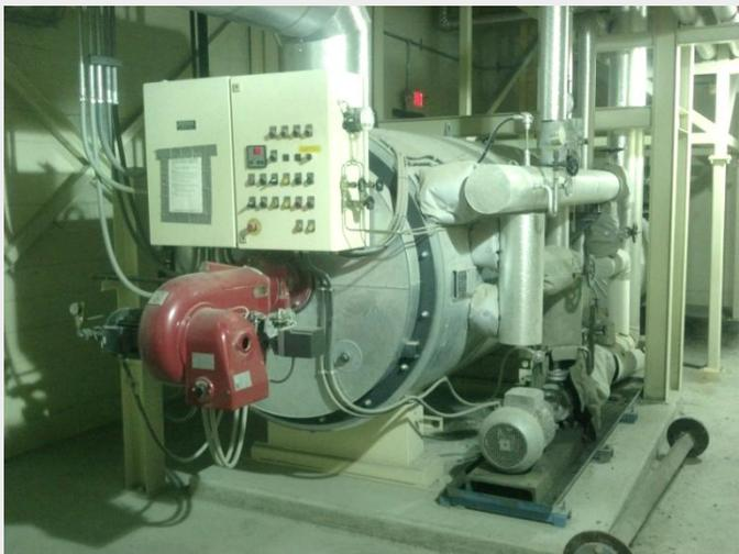
Heating units may be small enough to fit in a closet, or in the case pictured above, the units may be full-sized boilers that are installed within fire-rated isolation rooms. These rooms are typically diked to contain an oil spill and may be equipped with a self-contained fire suppression system. Note the excellent housekeeping, which is a necessity to prevent fire extension in the event of a leak.
