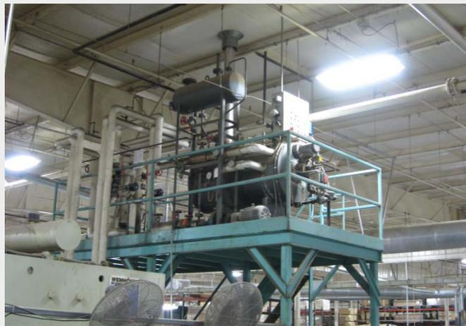
Shown above is a relatively small buffer tank with the expansion tank above. This particular unit is being used on a small plywood lamination press. Some systems may use as little as 20-25 gallons, while others may use thousands.
